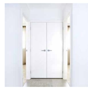
**Linen cupboard doors to match** High hollow core Hume flush panel with painted finish to linens (match internal doors).
