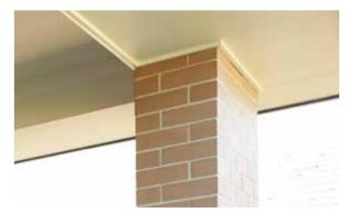
450mm fibre cement eaves lining
